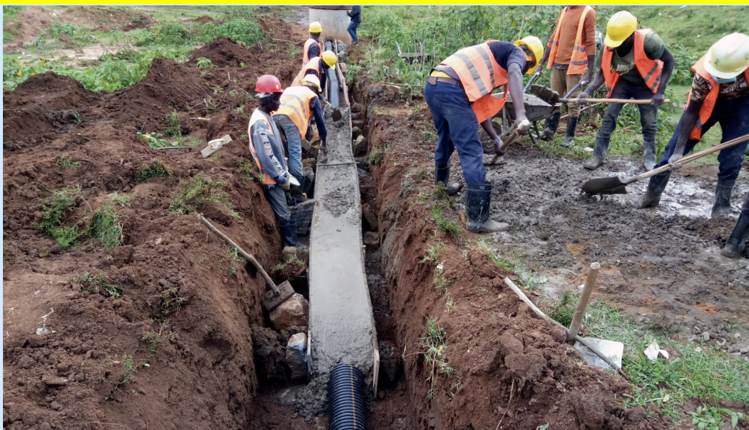
Haunching sewerline in Chepareria Hospital
