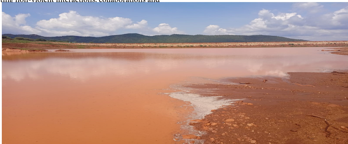
A section of Kasses Peace Dam on a rainy season.
