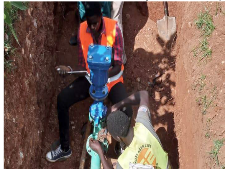
Installation of air valve along new water mains.
