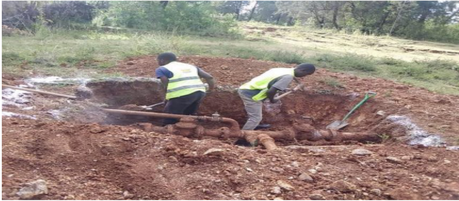
Exposing of existing water mains for rehabilitation.
