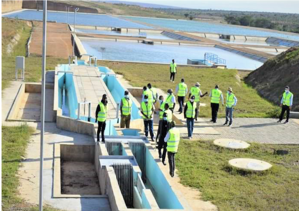
CRVWDA directors inspect the completion of narok town sewerage system
