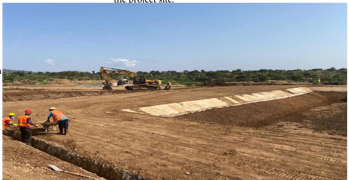
A section of Chepareria Town Sewerage
