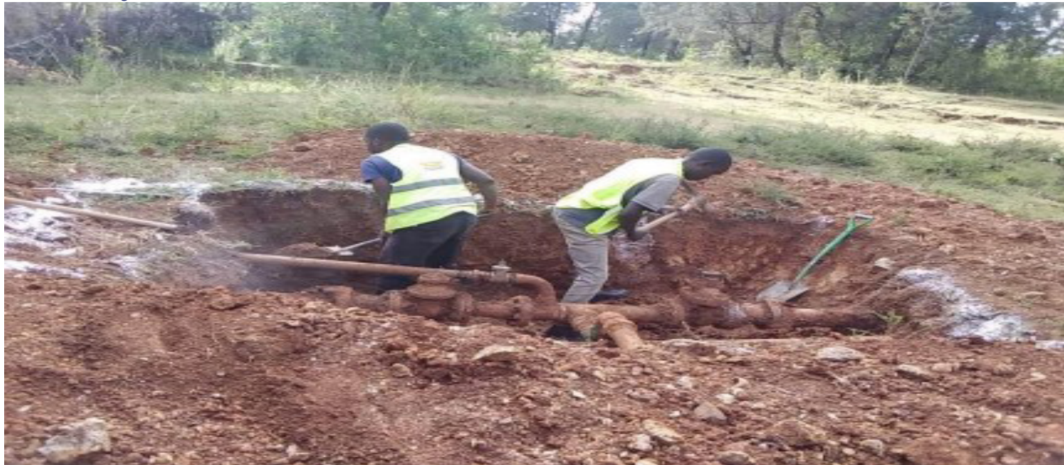
Exposing of existing water mains for rehabilitation.
