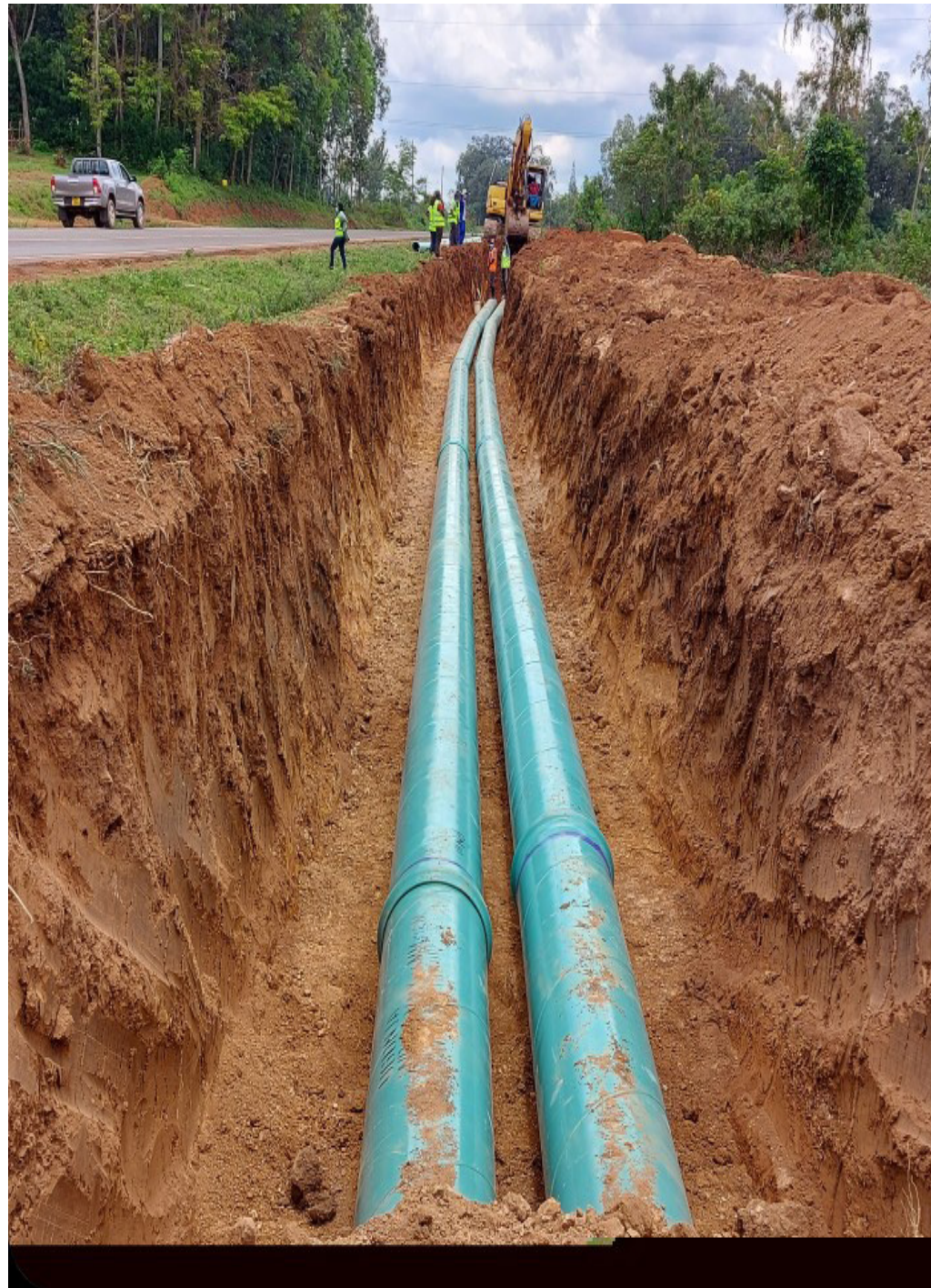
Laying of steel rising pipes
