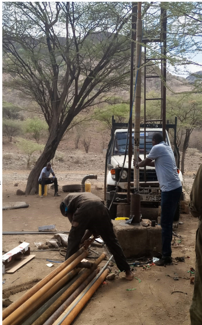
Replacement of kapau borehole mortar
