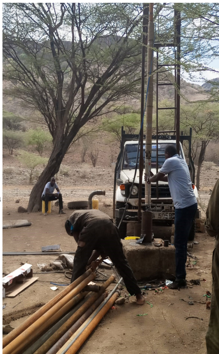
Replacement of kapau borehole mortar
