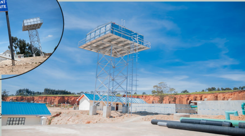
A section of Olkalou Water Treatment Plant
