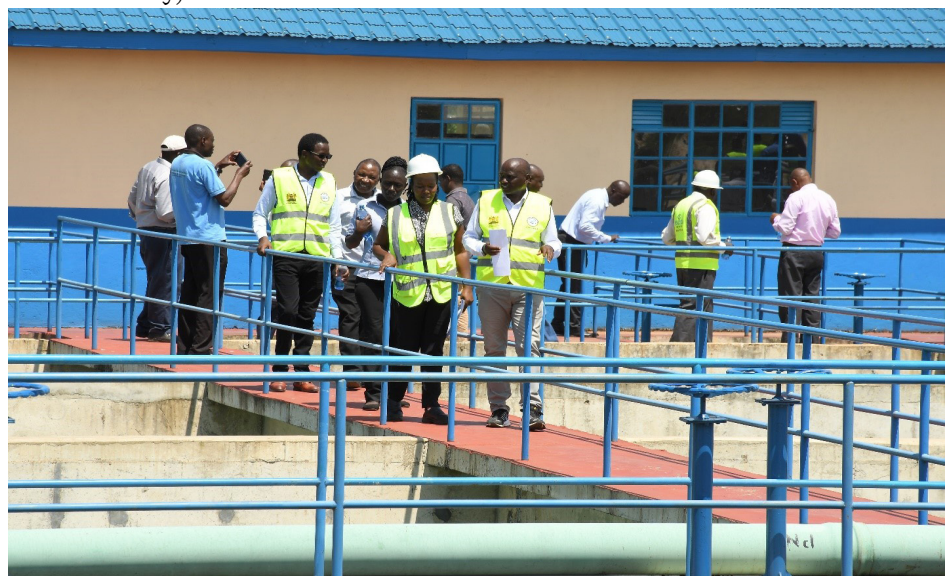
Inspection of Ugunja Water Supply Project, Treatment Works
