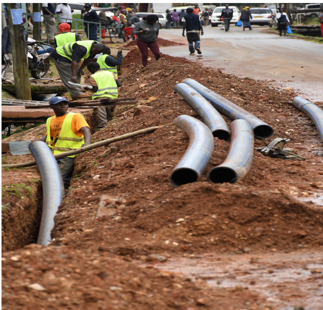
On-going laying of pipes in Kakamega Town.
