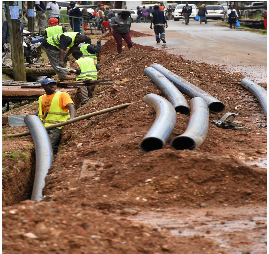
On-going laying of pipes in Kakamega Town.
