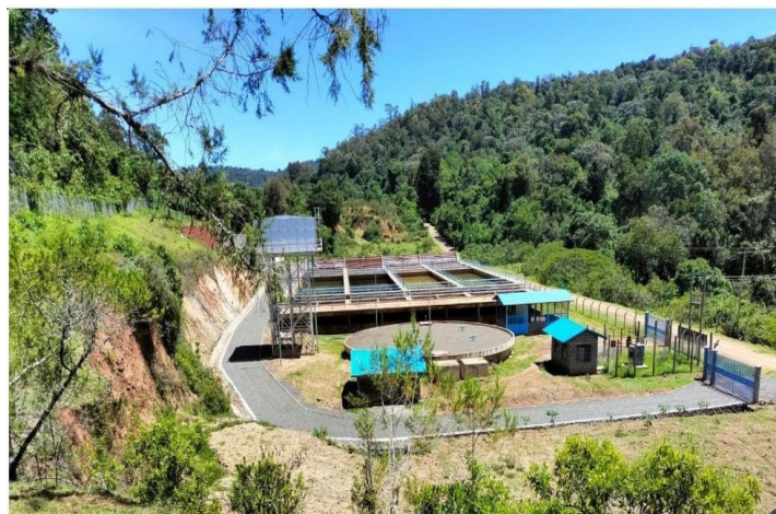
Chemususu Water Treatment Plant
